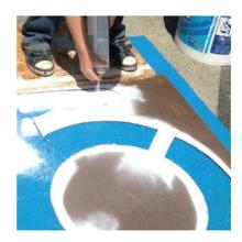
• It is recommended in California to paint a 4" white border to create a 49" overall size. Position the tape inside and outside the blue border creating the required 4" line.
