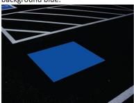
• After the blue square is dry, position the stencil again over the blue paint and spray the white for the wheelchair symbol.
